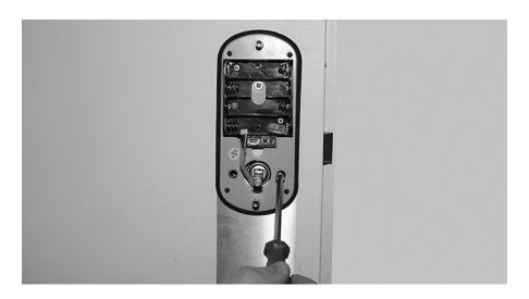
10. Connect the power cable. Adjust the cable so that it is not damaged by the square spindle. Put inside AA  $4 \times 1.5V$  batteries (K).
