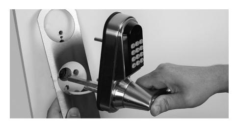
In some situations, when the front part of the lock can't be installed due to the lack of certain recesses, it may be necessary to re-drill the holes of the mortice lock. The spacing of the factory-prepared recesses may differ slightly from the spacing of the bushes in the front part.
