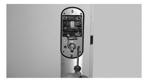
10. Connect the power cable. Adjust the cable so that it is not damaged by the square spindle. Put inside AA 4 x 1.5V batteries (K).
