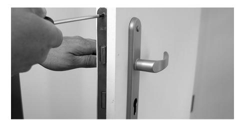
4. Try the inner part of the new lock (C) and mark the holes to be drilled (No. 1, 2). Remember to keep the cover straight. Then rotate it 180 ° and mark another hole (No. 3) that will help you to move the power cable to the other side of the door.
