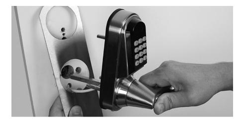
In some situations, when the front part of the lock can't be installed due to the lack of certain recesses, it may be necessary to re-drill the holes of the mortice lock. The spacing of the factory-prepared recesses may differ slightly from the spacing of the bushes in the front part.
