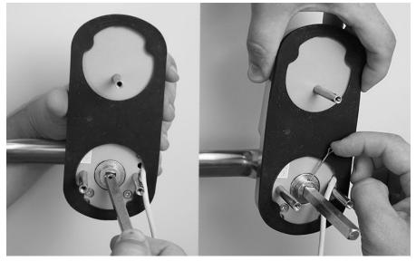
8. Fix the front part of the lock (A) with the metal sheet (E), inserting it into the mounting holes. Make sure that the cable connecting the control panel (A) and the power section (C) is correctly threaded through the hole.
